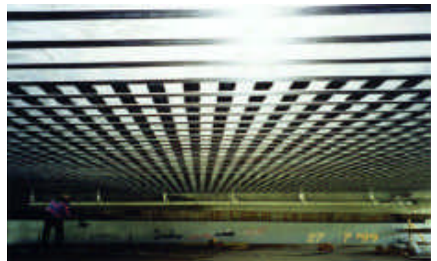
Fig 18 Applied CarboDur plates
