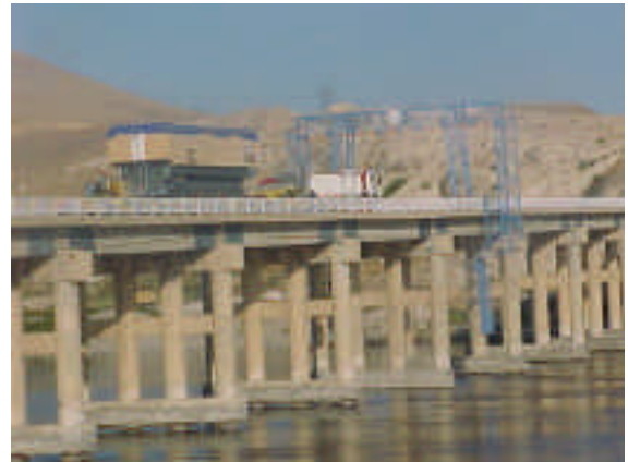
Fig 24 Heavy Transport on Karababa Bridge
