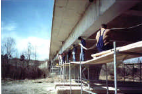
Fig 11 B7 Application on site
